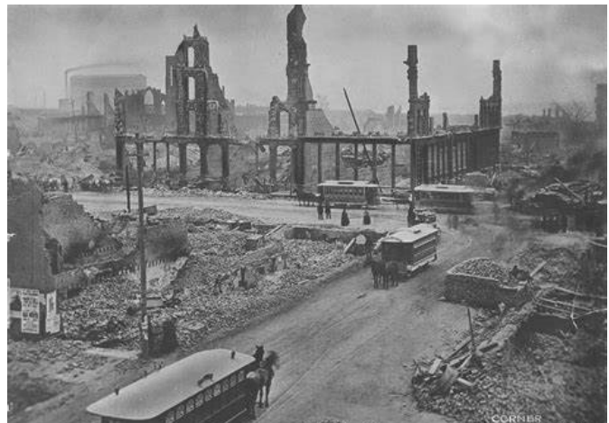
The aftermath of the 1871 Great Chicago Fire which burned 2,112 acres and left one in three Chicago residents homeless.
