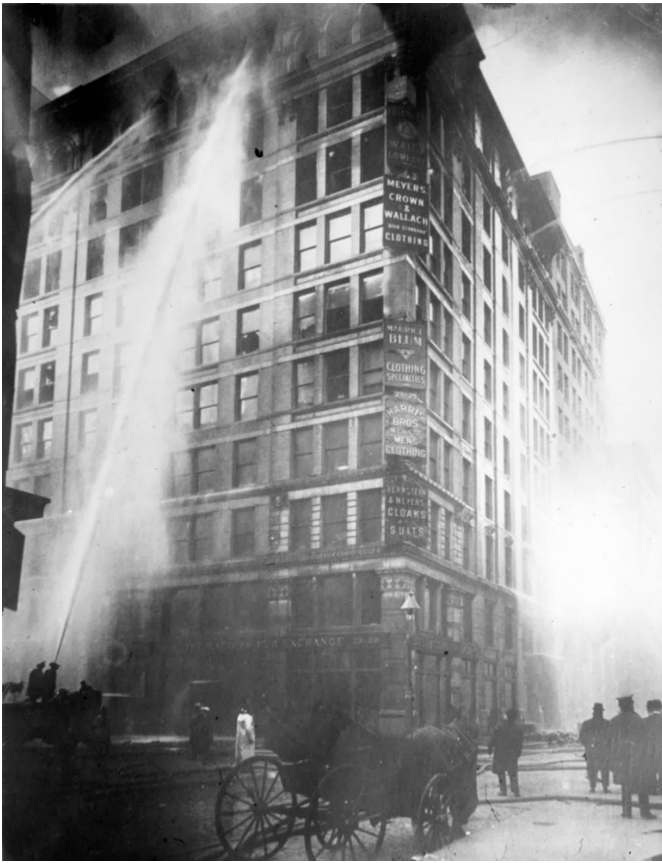
The 1911 Triangle Shirtwaist Factory fire in New York killing 146 people. After the fire new laws mandated better building access and egress, fireproofing requirements, the availability of fire extinguishers and the installation of alarm systems and automatic sprinklers.
